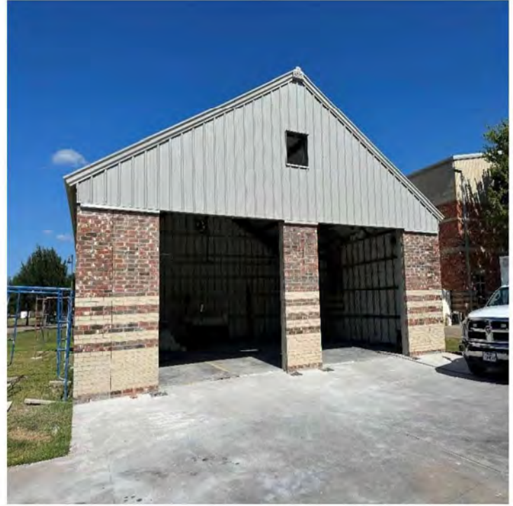
In Progress Building Enclosure
