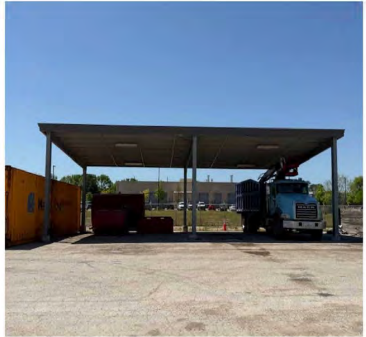
Road & Bridge Station, Crabb Texas
