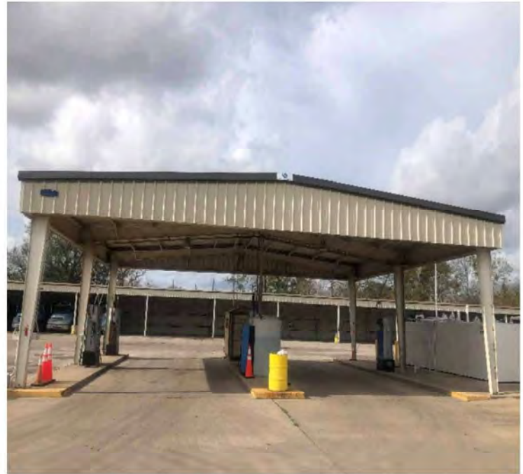
Canopy After Repair
