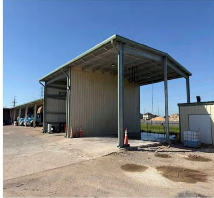
Wash Bay After Repair
