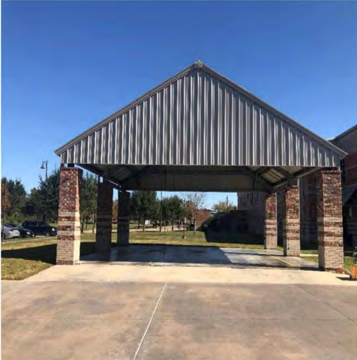
Building Before Enclosure
