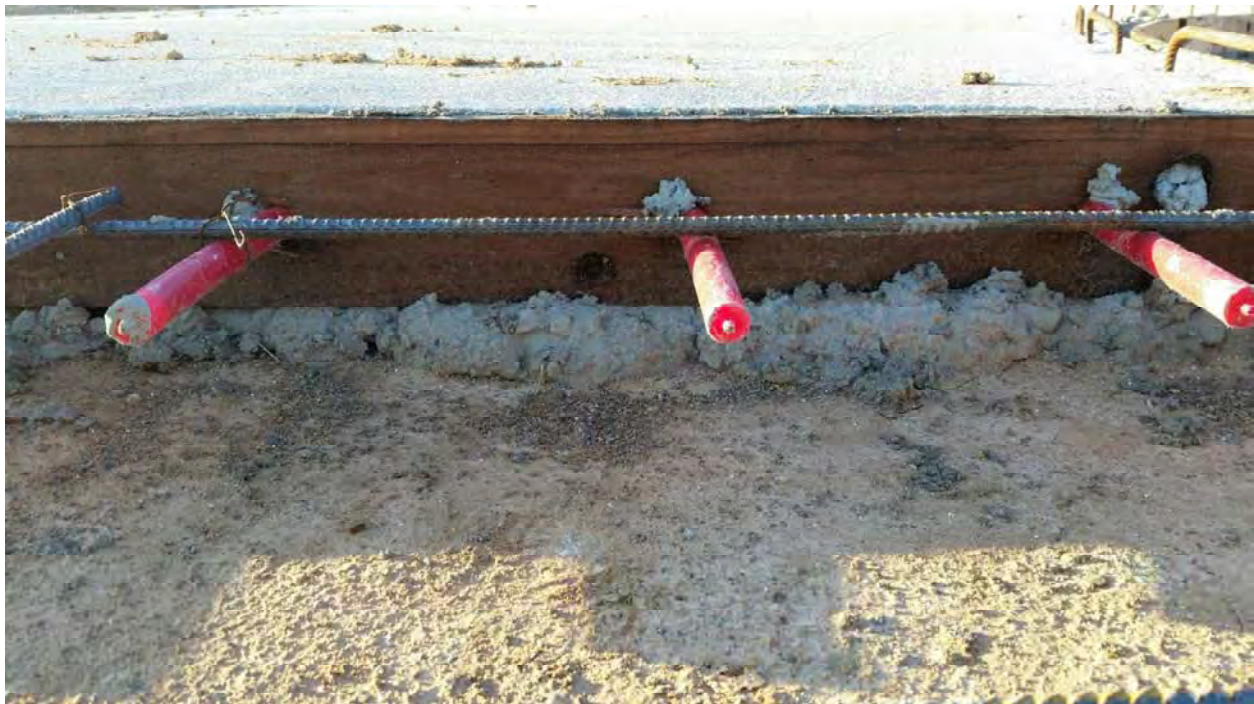
Image 8 - Concrete under headers at expansion joints does not allow expansion to occur correctly.
