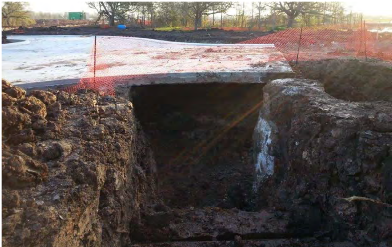
Image 14 - Excavation under or near pavement
