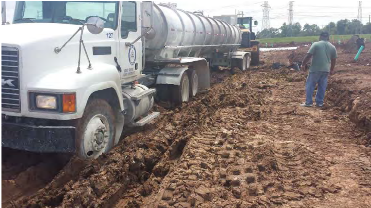
Image 7 - Possible deficiencies in subgrade and base include: Inadequate proof rolling or improper mixing of lime for subgrade, not extending lime mixture to edges of proposed limits of the stabilized subgrade, calculating lime for a 6 inch subgrade and mixing it 8 or more inches deep.
