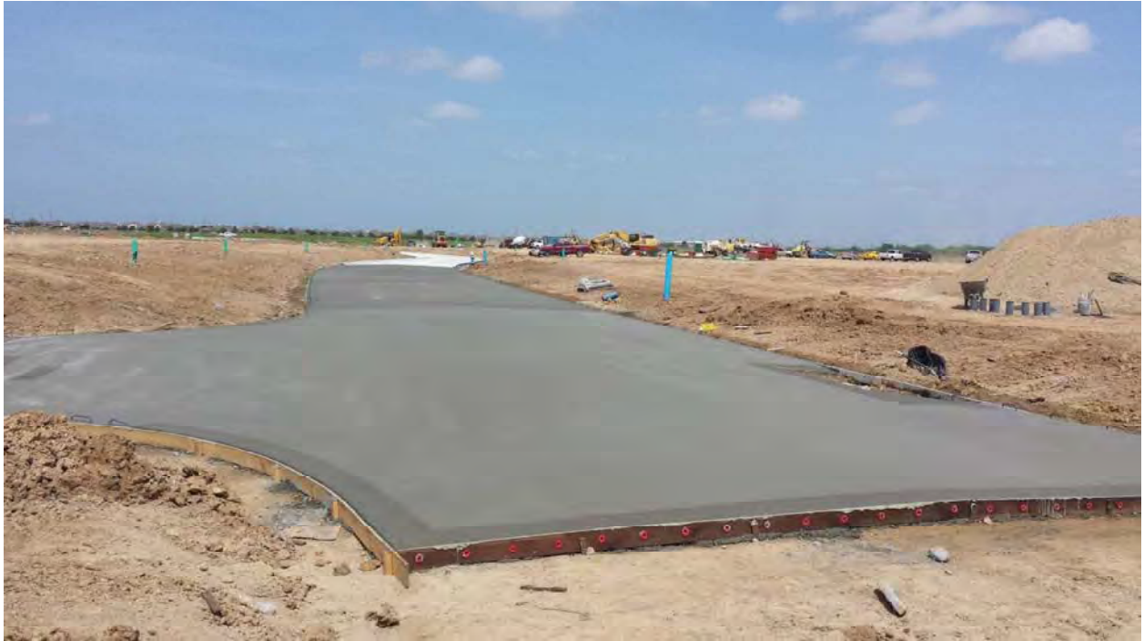
Image 11 - Membrane curing compound not applied to pavement
