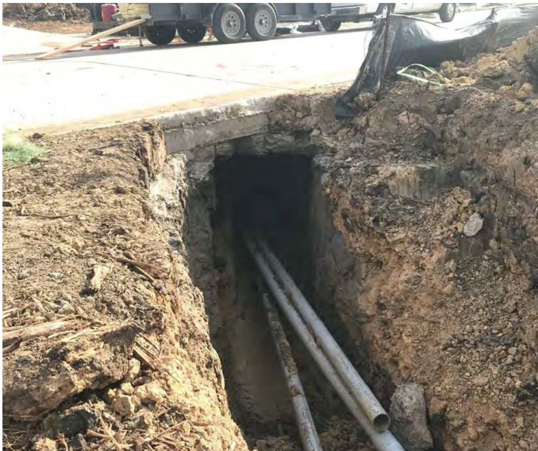
Image 18 – Private utility excavation beneath pavement
