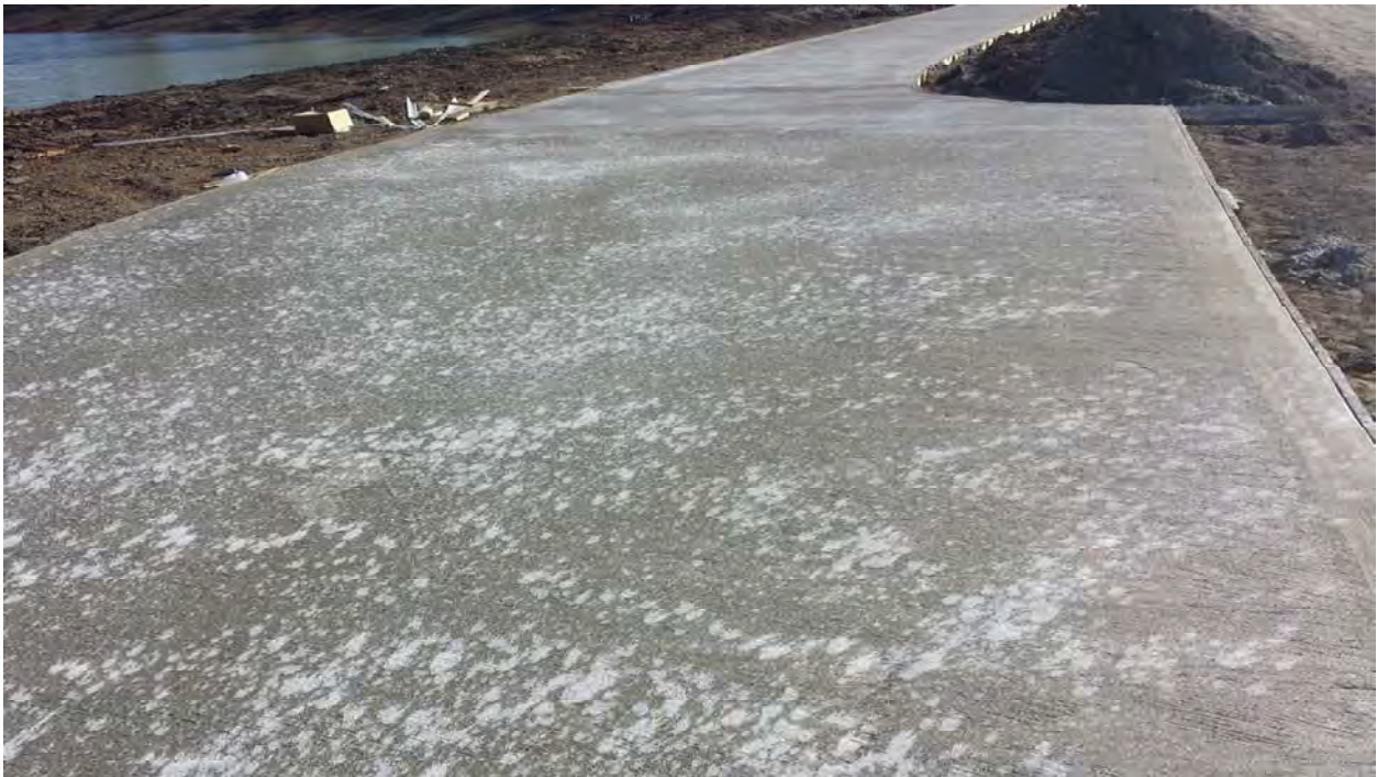
Image 12 - Inadequate curing compound
