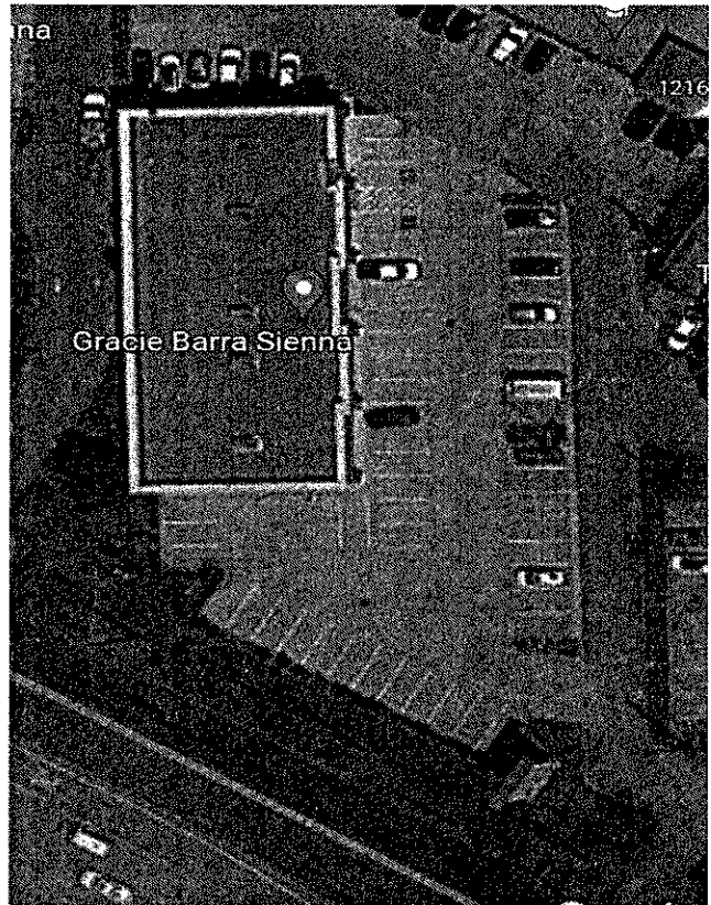
AERIAL VIEW - COMPLETED
