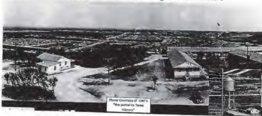
Figure 2 water tower at Camp Bowie 1940's (potentially one at Higgins or Needville)
