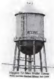
Figure 1 Higgins Water Tower of same origin as Needville's
