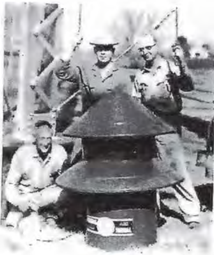
Figure 10 Needville Tower Whistle prior to installation
