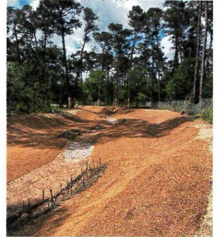
Stream construction photo from April 2021
