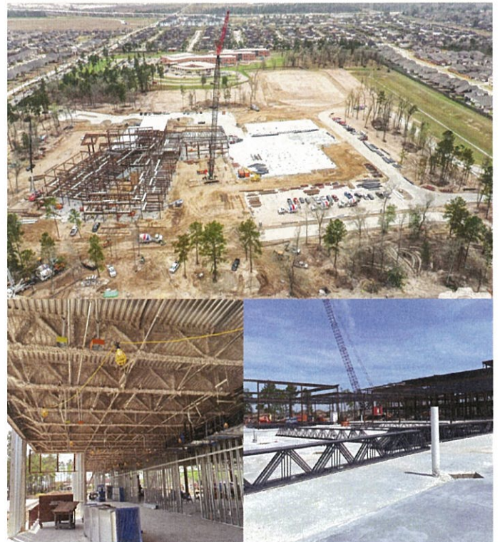
Humble ISD Middle School No. 10 Steel Erection.
