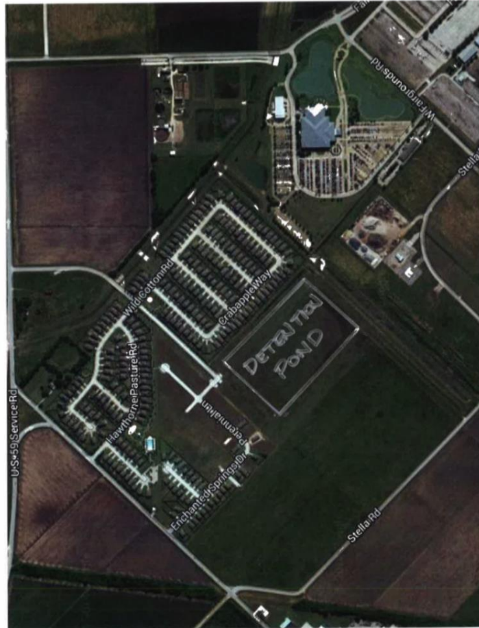
Figure 5 – Site Aerial Image
