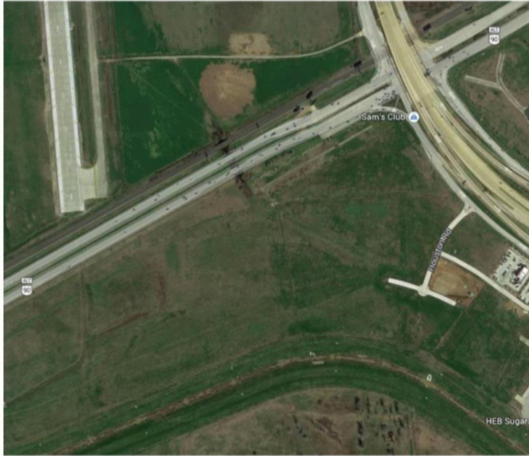
Figure 10 - Site Aerial Image
