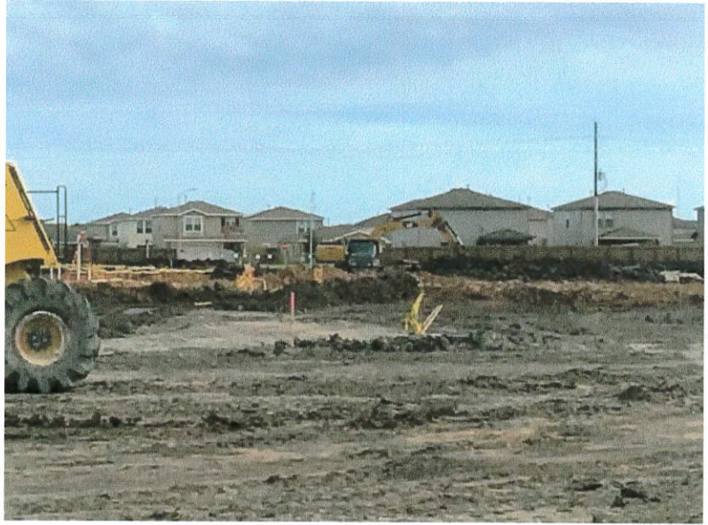
Burnside hauling off excess dirt
