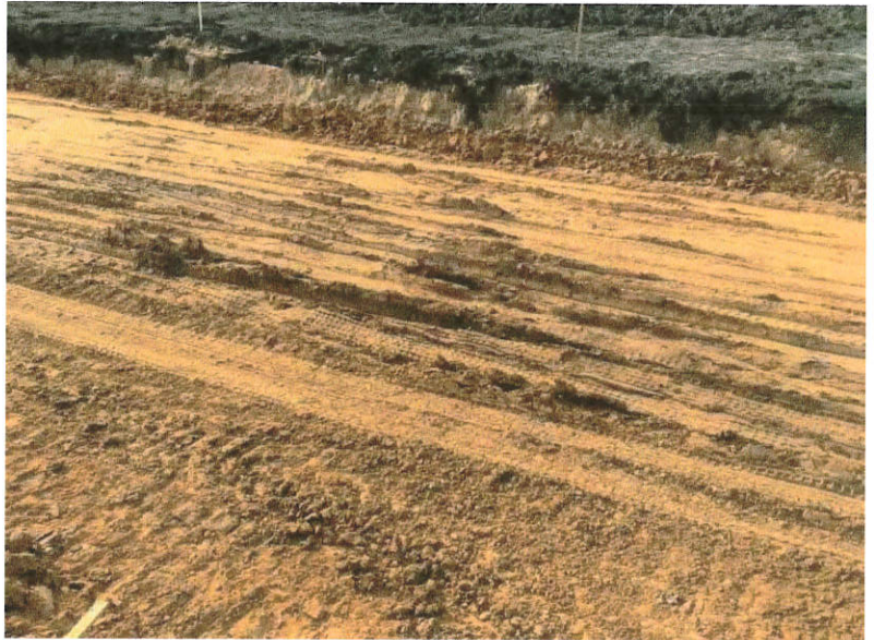
Fuel and Wash Bldg. pad. Burnside starting to place 2nd lift of select fill
