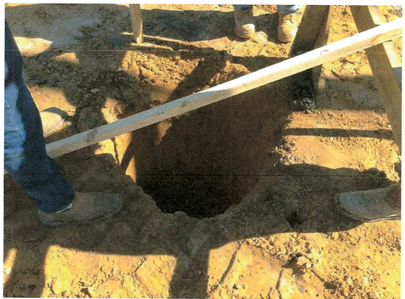
Administration Bldg. pier location all pier shafts measured 12' depth.
