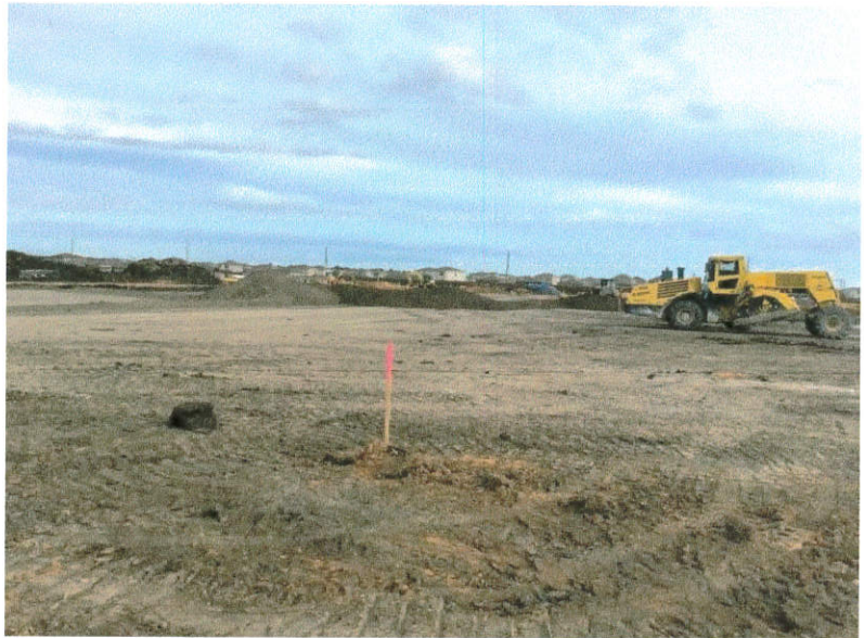
Bus Parking Lot area final grading and possibly reinforcement steel on 11/18
