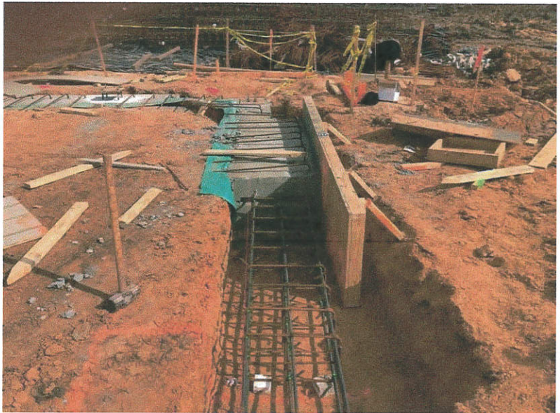
Joslin removing forms from grade beams poured 11/16
