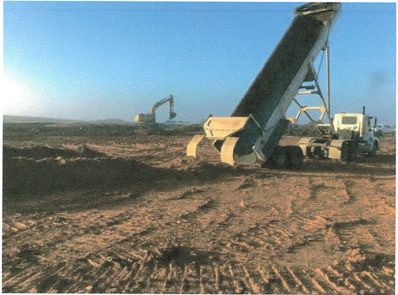
Maintenance Bldg. 4th lift select fill
