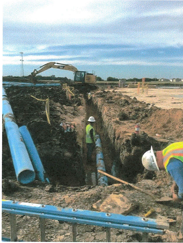
Installing 10" FL out to meter location.
