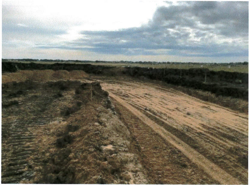
Fuel and Wash Bldg. pad. Burnside starting to place 2nd lift of select fill
