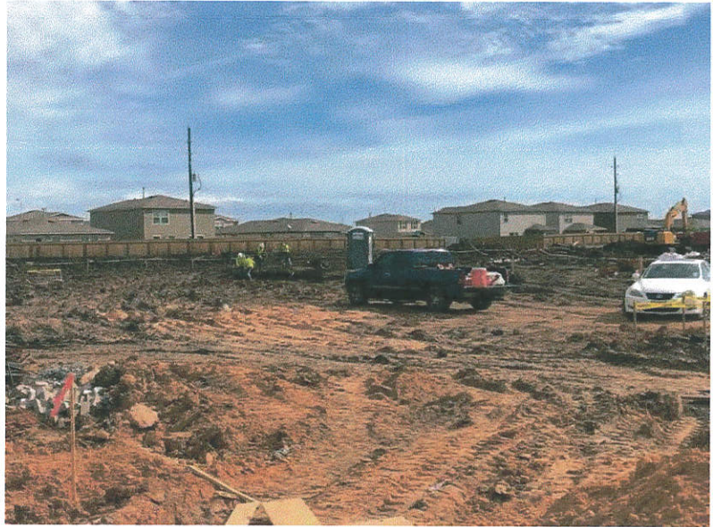
Joslin tying reinforcement steel for grade beams
