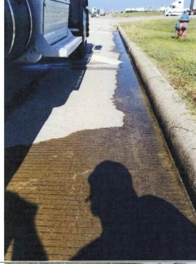
5-24-18 Photo 2 Soil containment stopped diesel from entering the storm drail.
