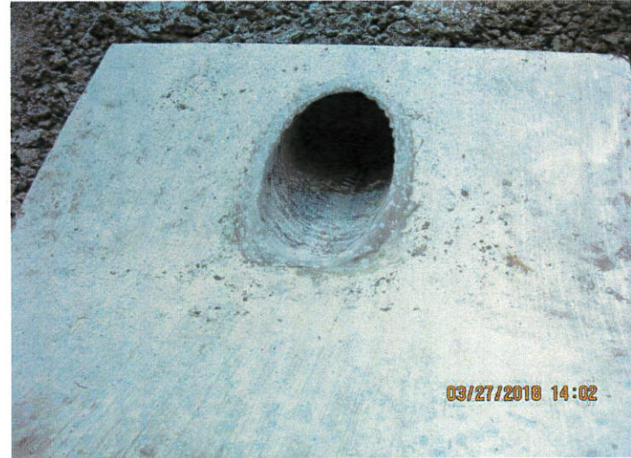
Looking West on the Ditch Showing 30-inch Outfall CMP
