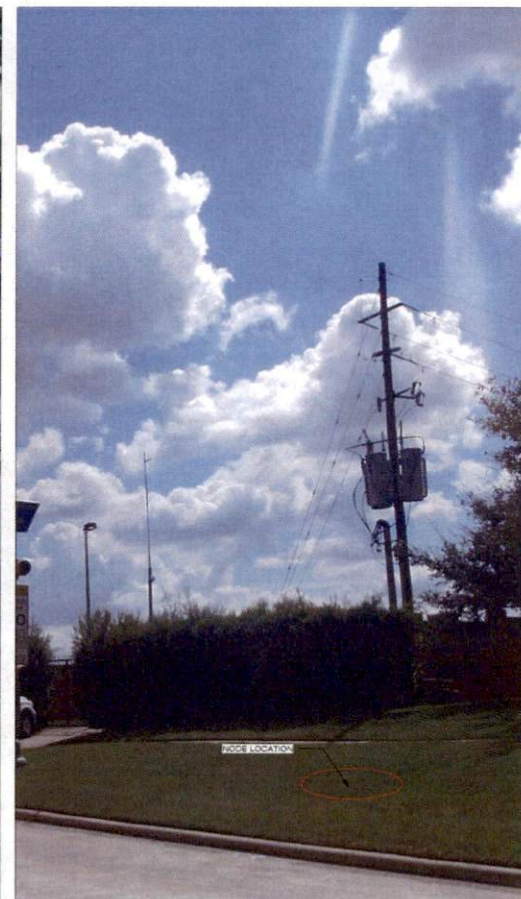
SITE PHOTO (EXISTING)
