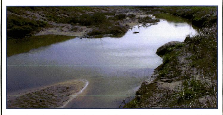
Reference Stream Segment: Note previously completed segment of new floodplain creation on Big Creek building a point bar (as a bench), with hydrophytic species colonizing it providing erosion resistance. Shown is creation – by stream building processes - of sinuous streambed by widening and curving into small floodplain. Also note a small backwater pool is forming in center foreground.
