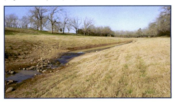
Small Weir-And-Pool: Previously installed by Applicant on Fulshear Creek some years ago to control head cut traveling upstream (out of sight behind camera position). Note long, gradual tailrace behind weir that moderates hydraulic jump and prevents scouring a pool below. Rather than scouring a pool below the weir, another pool would be dug in below weir to accept remaining energy flowing downstream.
