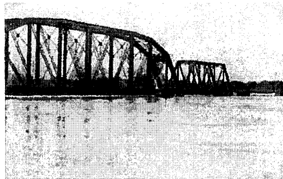
Flood waters at Brazos River Bridge
