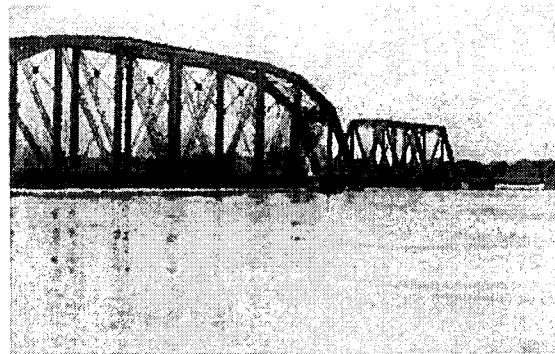
Flood waters at Brazos River Bridge
