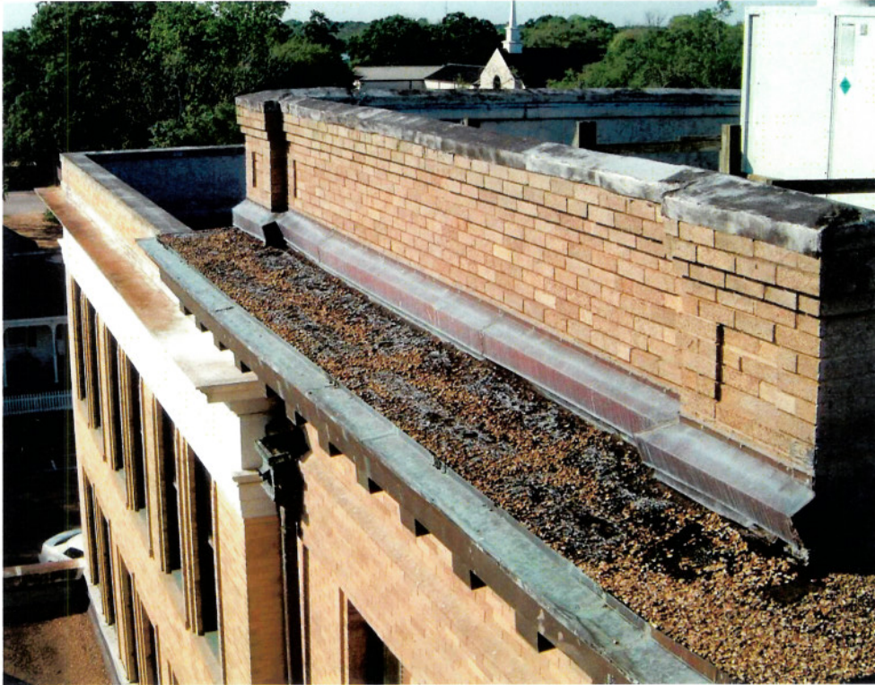
Membrane flashing over masonry caps
