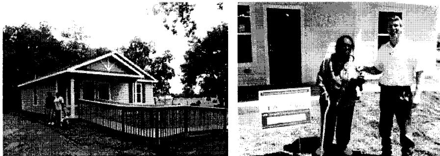
Reconstructed homes Tegrity has recently completed (HGAC Program)
