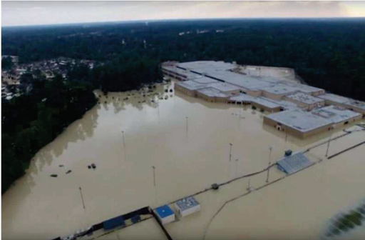
Harvey Flooding at Kingwood High School
