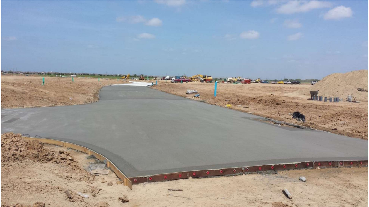
Image 11 - Membrane curing compound not applied to pavement
