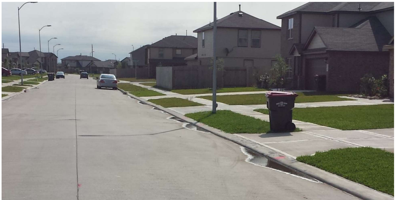
Image 4 - Bird baths which are relatively small in length, width, and depth do not require pavement replacement or lifting. Allowable width is approximately 12 inches.
