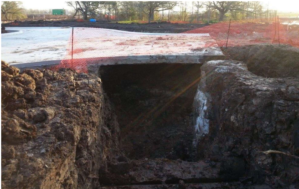
Image 14 - Excavation under or near pavement
