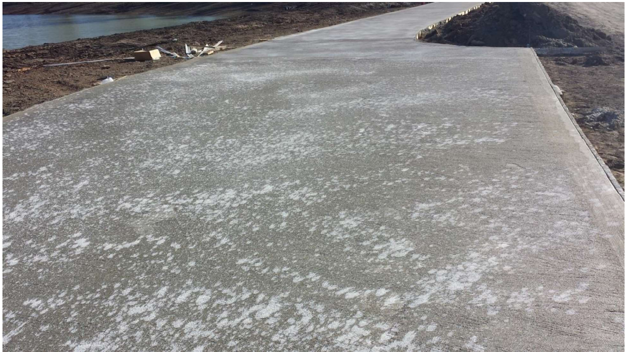
Image 12 - Inadequate curing compound
