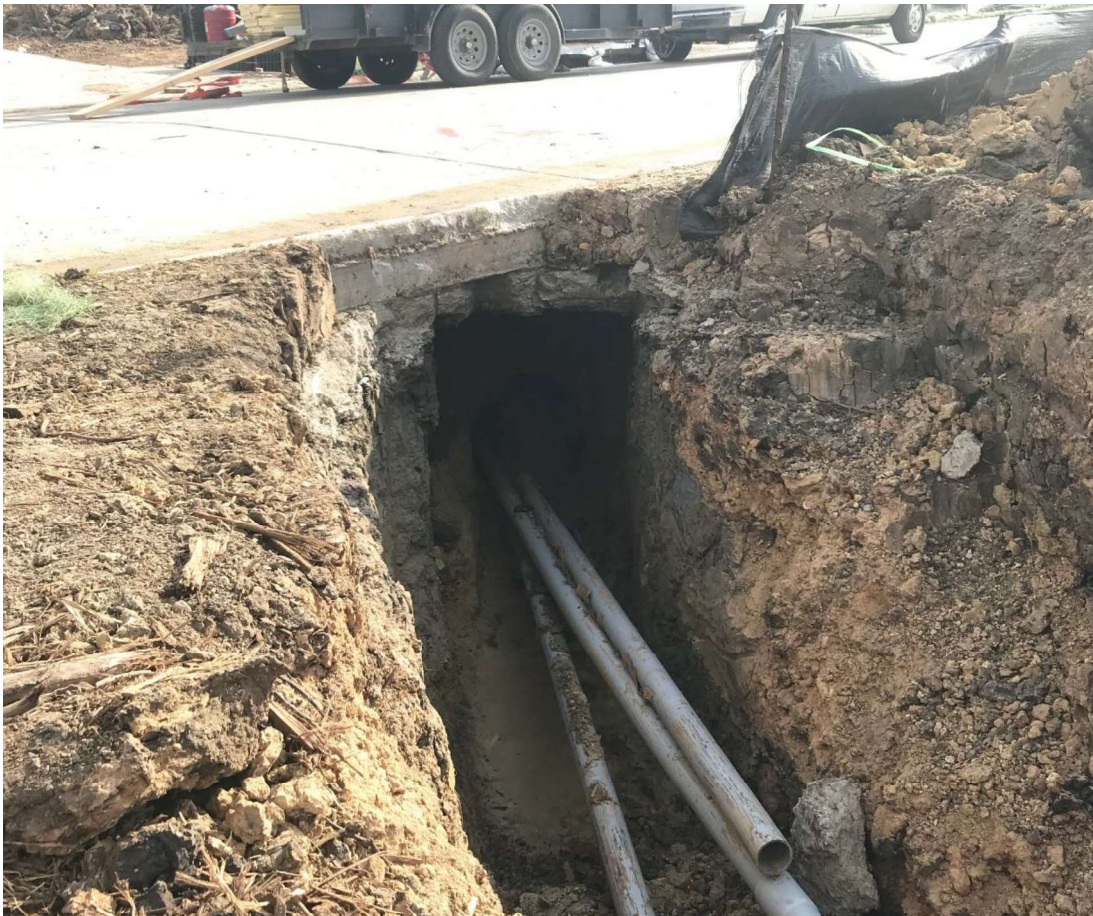
Image 18 – Private utility excavation beneath pavement
