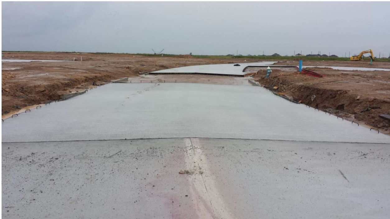
Image 15 - Not saw cutting within specified time (photo shows 4 day old concrete with no sawcuts)
