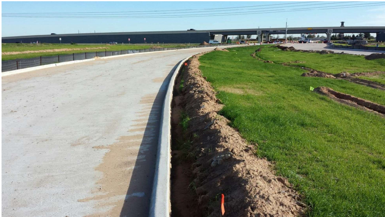
Image 13 - Silt fence or irrigation is placed directly behind curb cuts through subgrade and impacts lateral support.
