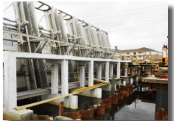
CITY BARN PUMP STATION BAR SCREENS - HMGP FUNDED
