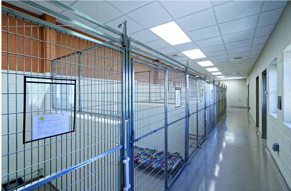
Attractive Kennels with bright lighting levels, epoxy floor finishes and sound absorbing ceilings make quiet, inviting public spaces.
