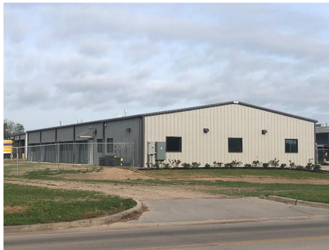
Building built in 2019 and designed by Shelter Planners of America
