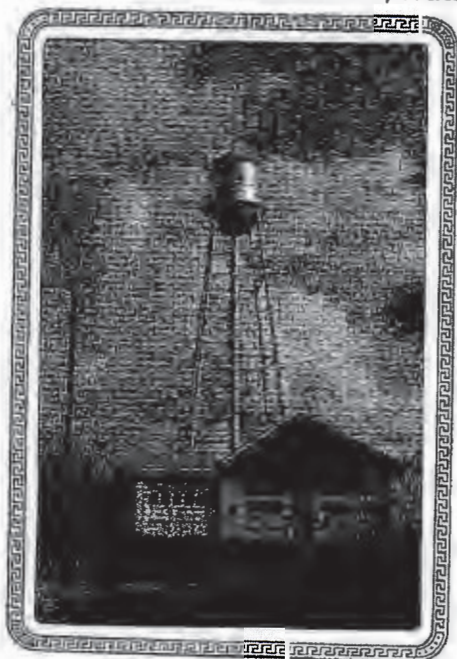
Figure 8 Firehouse prior to addition
