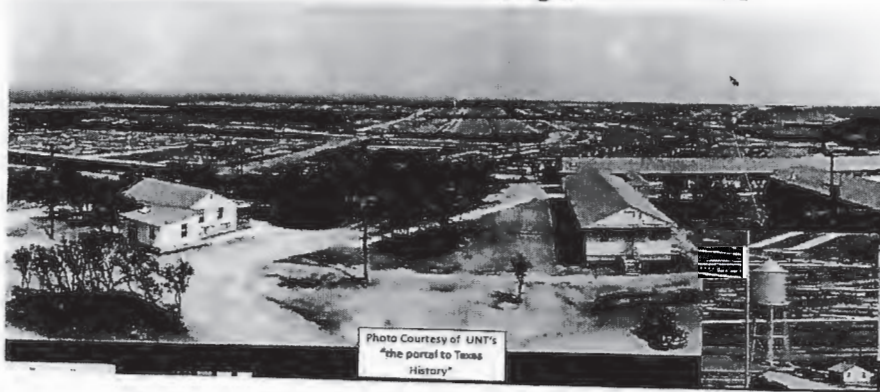
Figure 2 water tower at Camp Bowie 1940's (potentially one at Higgins or Needville)
