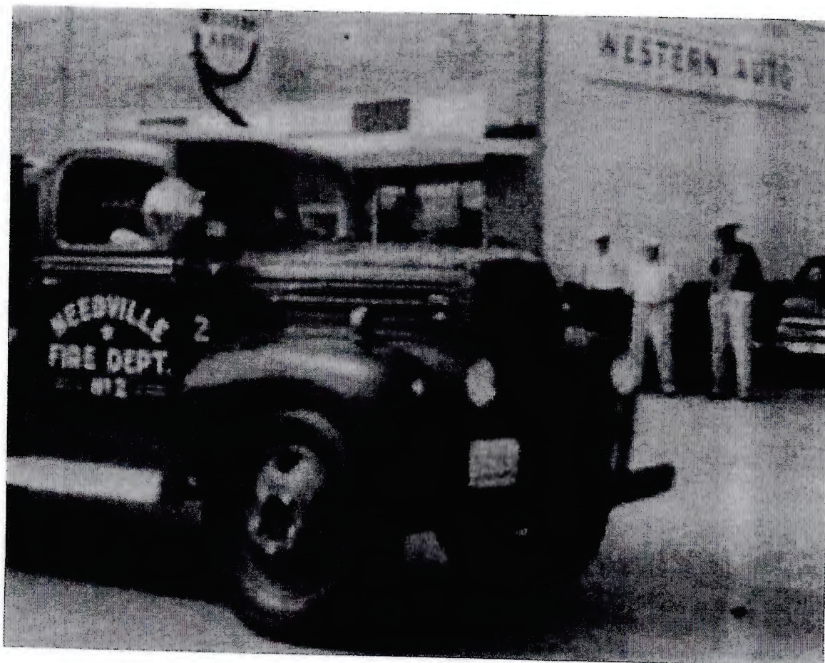
Figure 6: 1947 Pumper Truck, Still in Needville VFD possession
