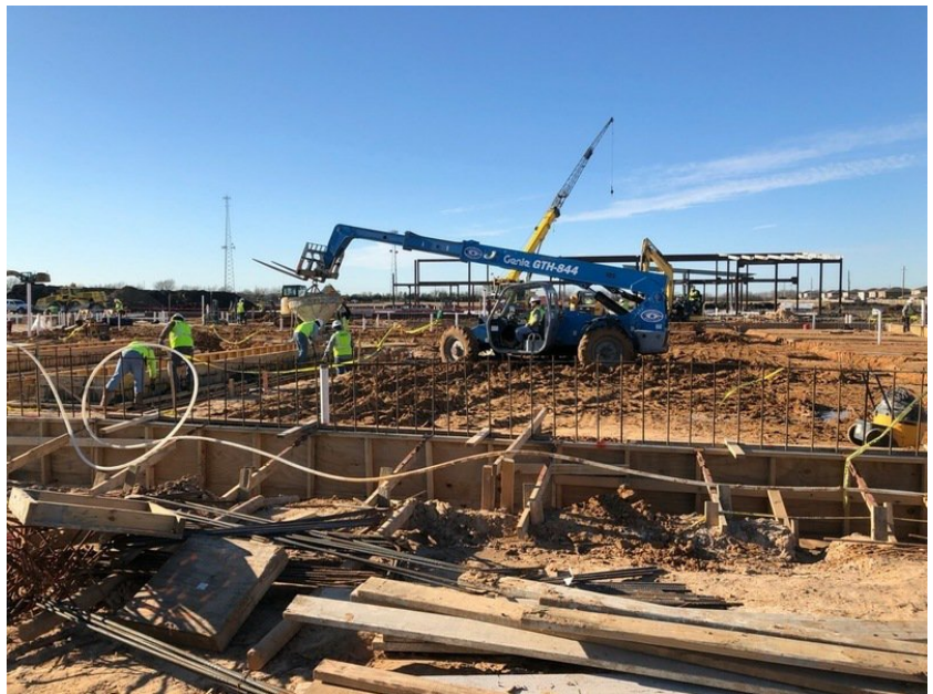
Pouring concrete in Maintenance building bus lift
