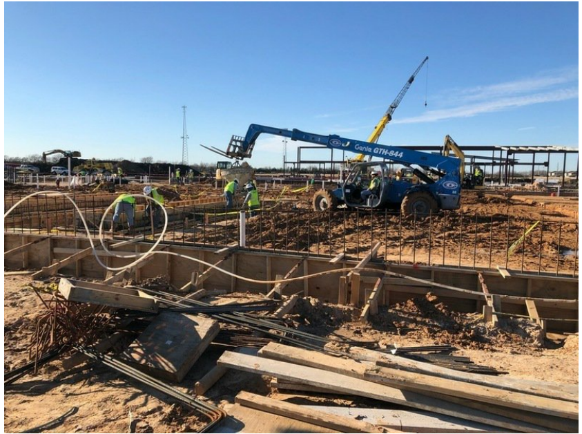
Cont- to poured in Maintenance building bus lift
