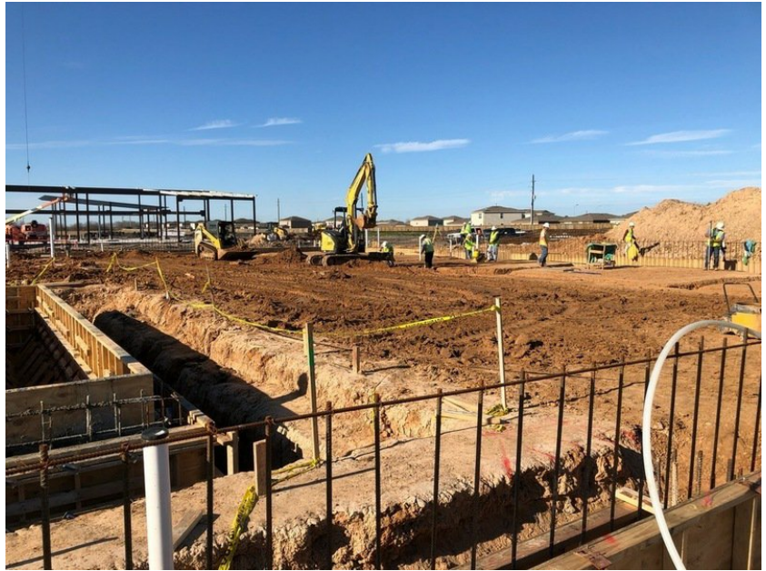
Joslin grading in Maintenance building
