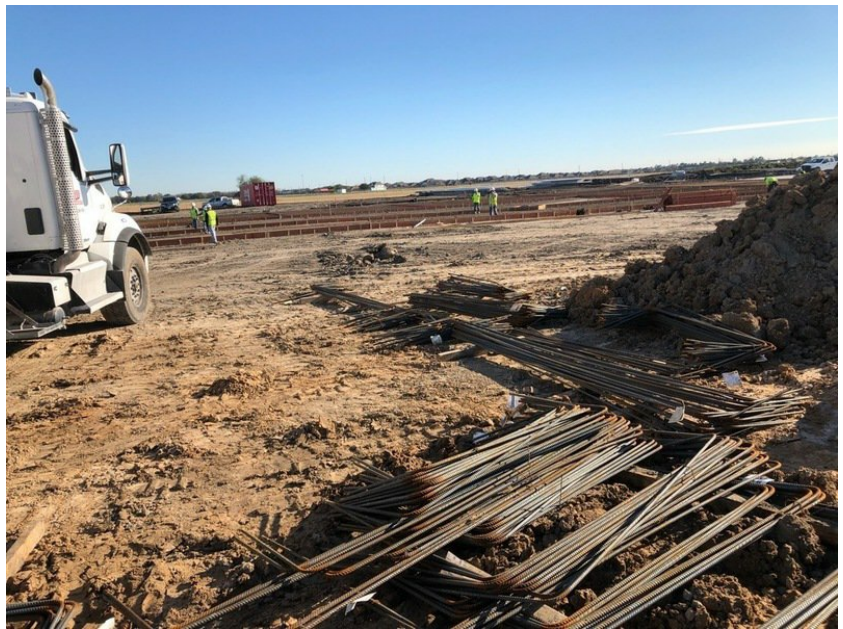
Joslin setting rebar
