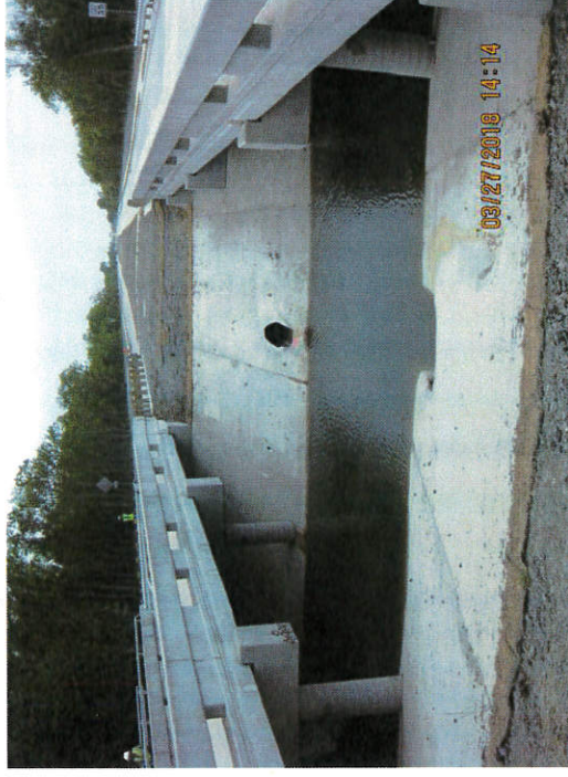
Looking West on the Ditch Showing 30-inch Outfall CMP
