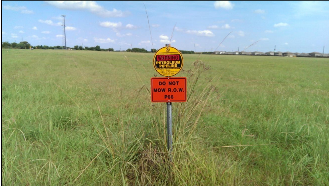
Photo 3. Pipeline marker on property.
